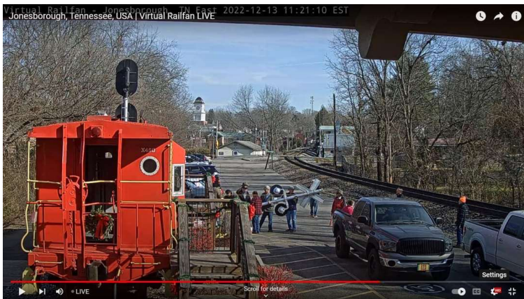
The crew unloading the crossing guard, ready for erection.
