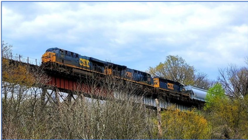
[Above] CSX northbound over Boones Creek Viaduct.
