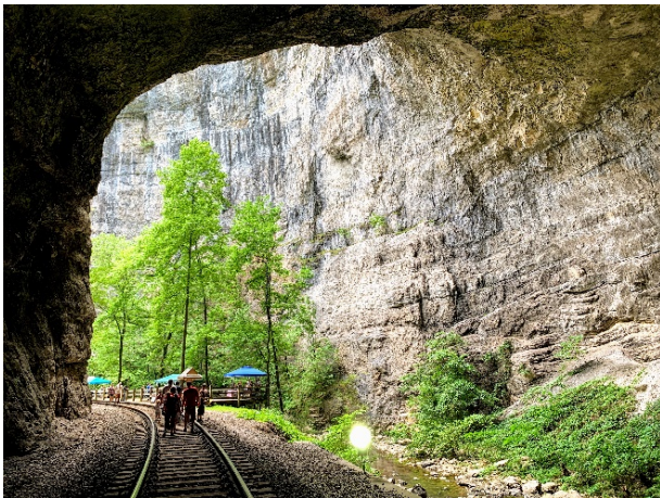
Looking from inside toward the front
