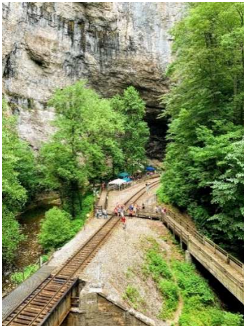
A bird's eye view at the east end of the Tunnel
