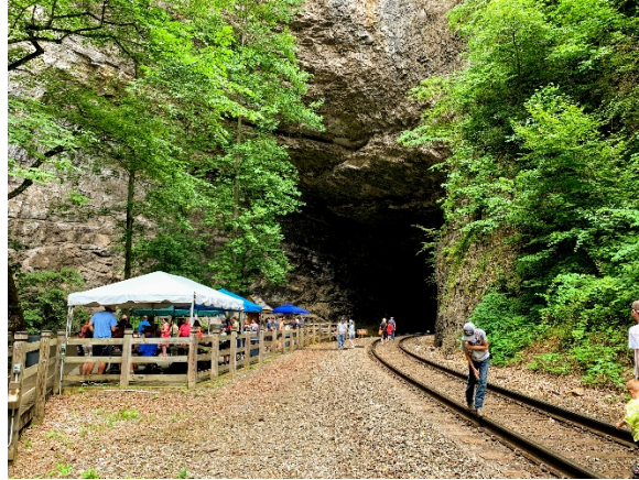
Ground view of the west end of the Tunnel
