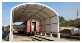
[report from "Turntable Times", Roanoke NRHS. Photo by Lewis Foster] Once the 512 was moved inside the car shelter, we began the process of removing the bottom edges of the side sheets to replace some extensive rust damage and expose the side sills of the car.
