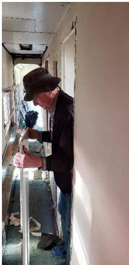
David Denny removing bedroom doors.
