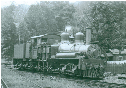
Marion and Rye Valley No. 1 at Fairwood, Va. allows you a good look at the unique design of the shay locomotive. The wooden cowcatcher is a nice addition to the locomotive, but where is the headlight?
